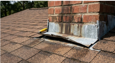
Roof-to-wall flashing
